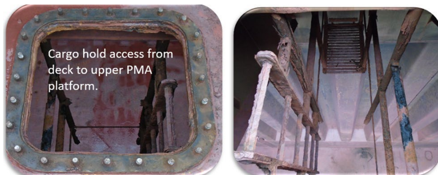
Figure 4: The deck access and upper platform on a 10-year-old vessel
