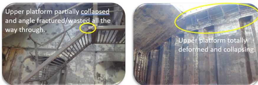
Figure 3: The deck access and upper platform on a 10-year-old vessel
