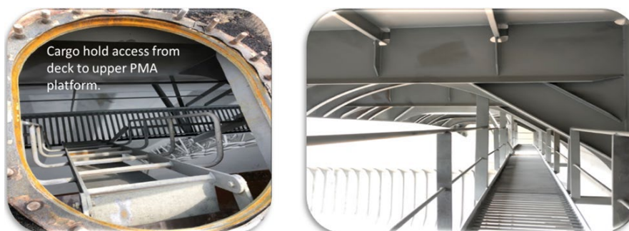
Figure 2: The deck access and upper platform on a 5-year-old vessel
