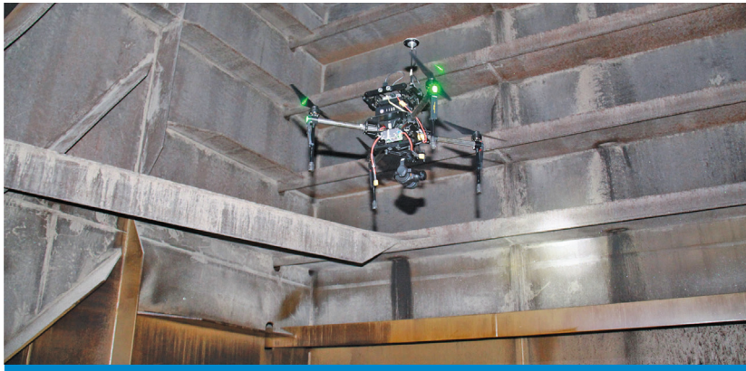
Remote inspection to internal structure through drone usage
